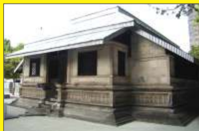
The Malé Friday Mosque, built in 1658, is oldest mosque in the Maldives, and is mostly constructed out of coral.
