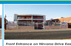
Front Entrance on Nirvana Drive East
